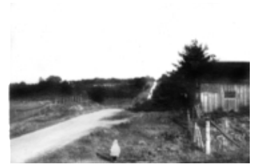
AFC 465-S1-I5 Commissioners Rd E [at] Wharncliffe [Road]. -- ca. 1905-1912. -- 1 b&w photograph (tiff, jpg)
