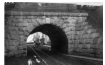
AFC 465-S14-I10 Thames Street subway. -- ca. 1905-1912. -- 1 b&w photograph (tiff, jpg)
