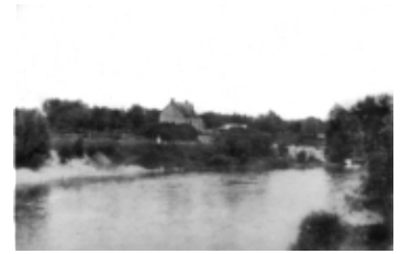
AFC 465-S1-I14 From Commissioners Rd across Springbank [view of house and barn across Thames River]. -- ca. 1905-1912. -- 1 b&w photograph (tiff, jpg)
